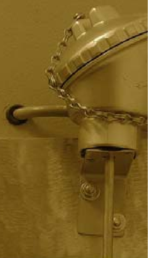
VALVE ROOM TCR-3. B1
